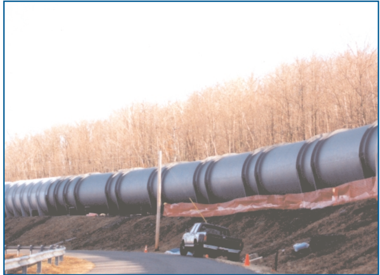
Silprocoat™ RTV coating on one of the largest water pipes in North America. This pipe, previously painted with lead based paints was coated with Silprocoat™ completely encapsulating the lead and providing a formidable barrier against corrosion.
