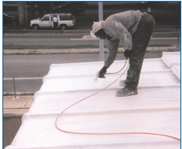
Because Midsun Silprocoat™ RTV Coating is highly water repellent, with built in adhesion promoters, it prevents electrolytic galvanic reactions from occurring.
